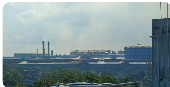
Fig. 11.6 Tata Steel's Jamshedpur works, India's oldest integrated plant still at work, beside the Subarnarekha.
