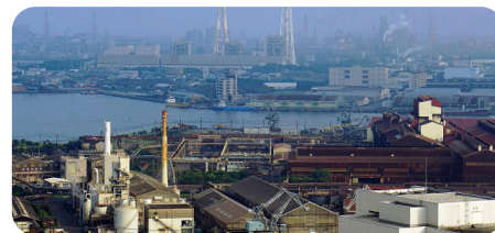
Fig. 11.19 Yawata works, Kitakyushu: Japan's first modern steel works (1901), on the shore of Dokai Bay.
