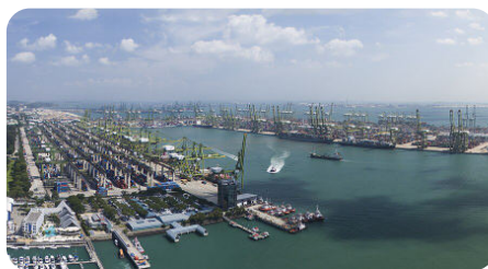
Fig. 19.12 Pasir Panjang terminal, Singapore, the world's leading transshipment hub.
