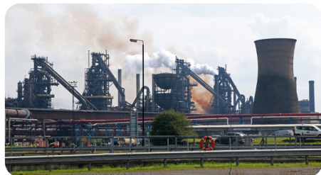
Fig. 11.2 Blast furnaces with their stoves and gas mains at an integrated works.
