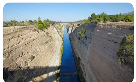
Fig. 9.20 The Corinth Canal, cut through rock walls up to about 90 m high.
